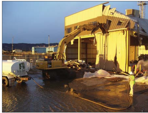
Gun Mole Pier Bldg Demolition, Hunters Point Shipyard
